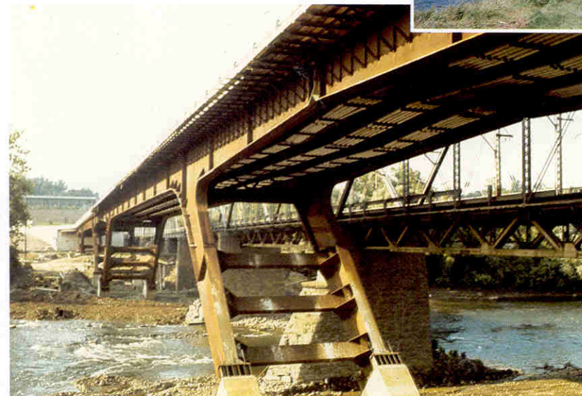
Bridge made of weathering steel
