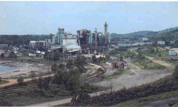
Plant recycling vanadium from spent catalysts
